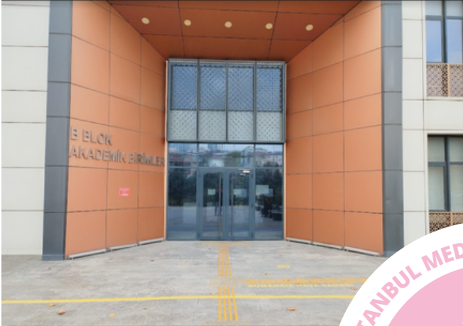
Tactile Ground Surface Indicators
