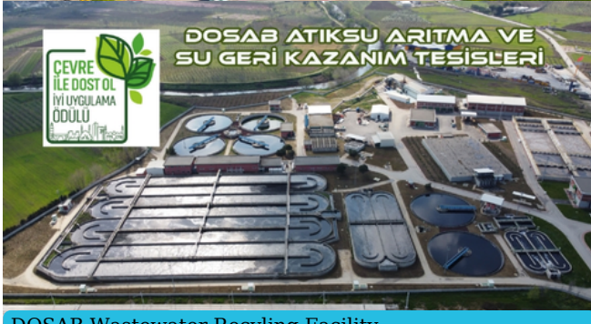
DOSAB Wastewater Recycling Facility
