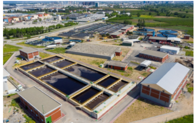
DOSAB Wastewater Recycling Facility
