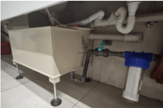
IMU Greywater Recovery System
