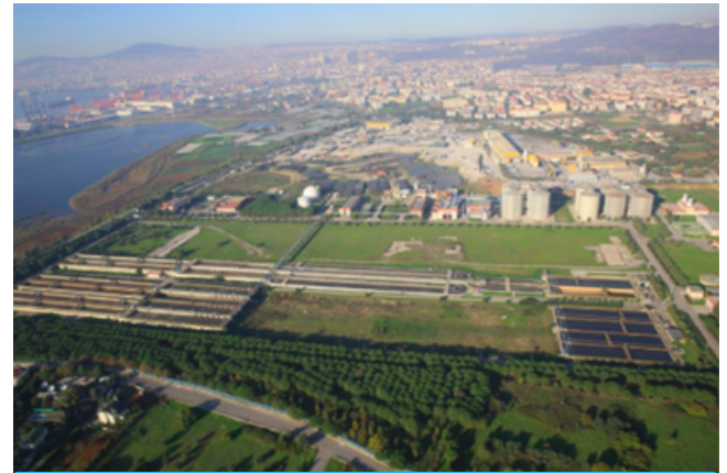
İSKİ Tuzla Advanced Biological Wastewater Treatment Plant
